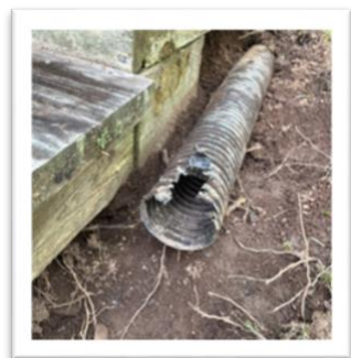
Image left: The dug trench and destroyed drainpipe.
