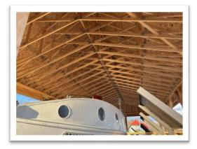
important is to face the OSB on the boat shelter gable ends with pine or cedar. OSB is a fiberboard and not suitable for long term exposure to weather. Site signage will be placed on the west gable that faces Marina Road.
