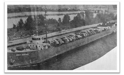
new cars on her deck. The boat was old, built in 1896, and was small by today's standards at 406'. She was powered by a triple-expansion steam engine that produced 2,000 HP. She was designed to tow a barge of about the same length, so was given extra horsepower.
