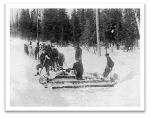
On the other hand, too much snow was just as bad and impeded both logging and railroad operations alike. In the logging camps men sometimes spent all night plowing the ice roads with wedge plows (image left) pulled by a large horse team. This had to be done so the water tank sleigh could sprinkle water on the road to freeze. A rut cutter then cut two ruts in the ice for sleigh runners which enabled large loads to be moved.
