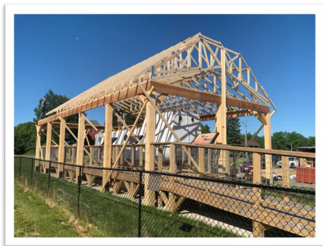
Framed and ready for roofing,
