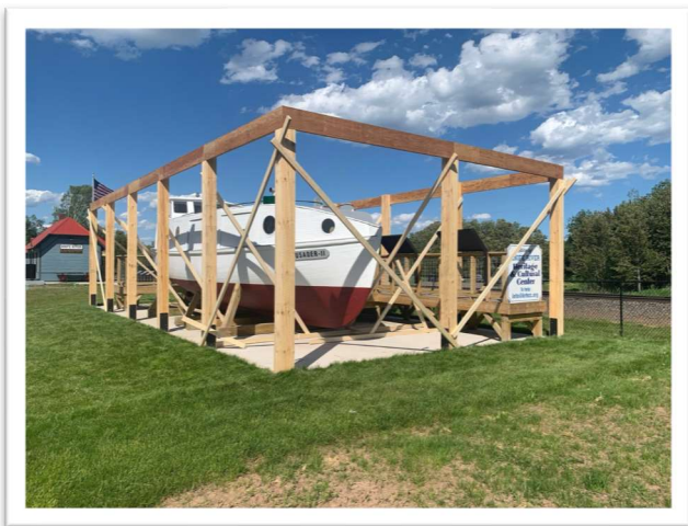
Supporting 8 x 8" posts in place
