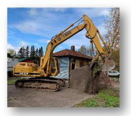
The skilled backhoe operators from Ostman Trucking & Excavating made quick work of carefully removing old depot apron. The space left was filled with Class 5. Photo: Paul von Goertz
