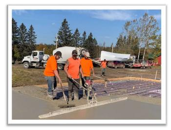
The mood was almost festive for the sidewalk superintendents who were present on October 21 to see 32 cubic yards of concrete poured to form the 23' x 46' commercial fishing exhibit slab. The concrete workers (photo left) from Primetime Concrete on Old North Shore Drive smoothed freshly poured concrete. Three truck loads were required. Primetime was good to work with, met our
