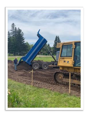
Image left: Slab footprint with sidewalk from interpretive displays to the slab. Image right: The dirt work required to bring slab to grade and serve as slab base required 100 cubic yards of clean coarse sand.
